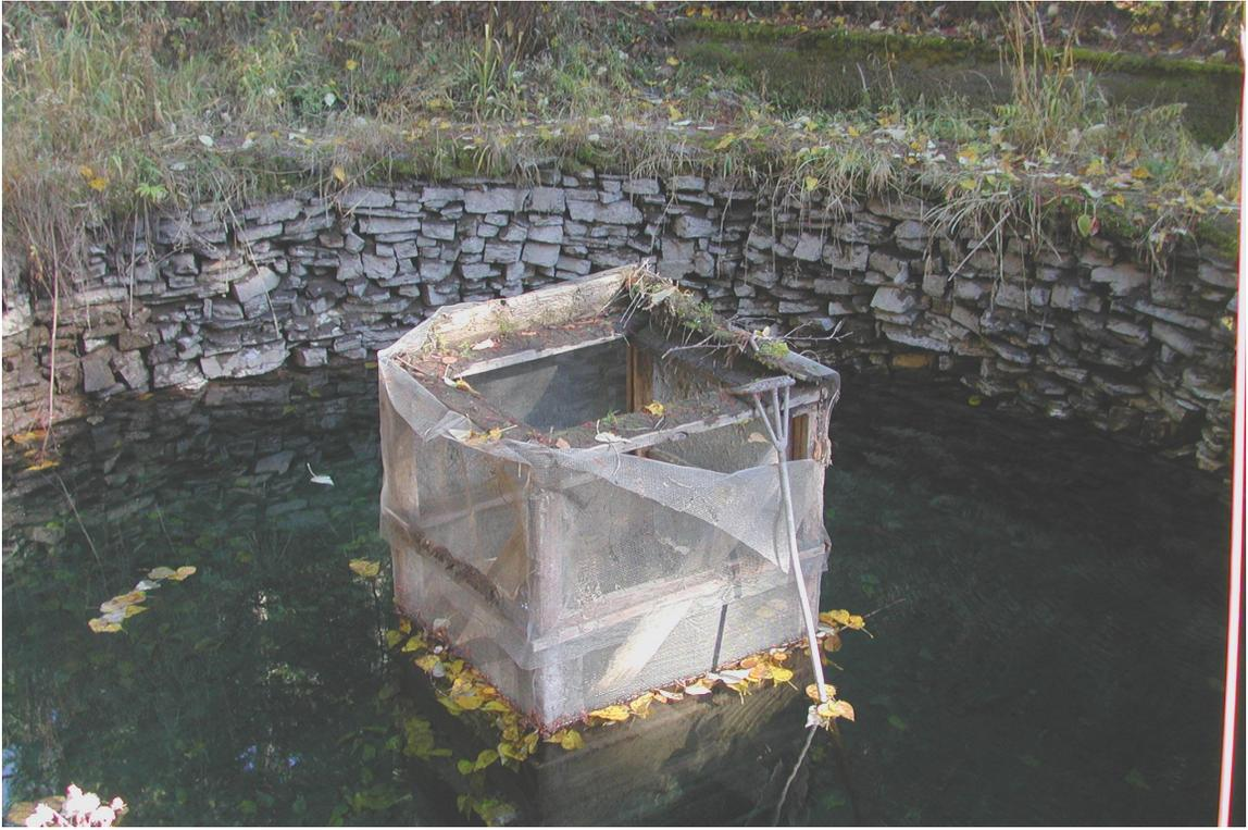
Figure 48. City of Troy water cistern O'Brien Creek, with old outlet pipe screen cover.
